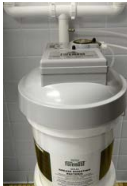
ATTACH TUBING TO FITTING
