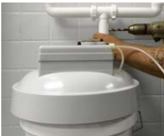
DRILL AND TAP DIRECTLY INTO LINE
