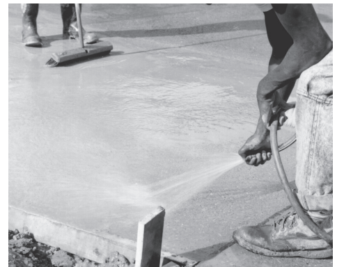
Top Surface Is Washed To Expose Aggregate
