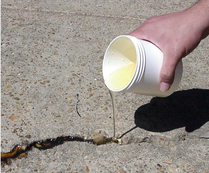
Repairs Joints In Concrete Floors
